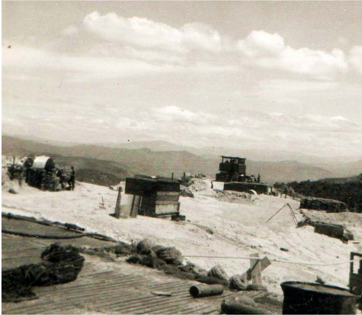
Cpl. Dwight Williams took this shot of what he seems to recall was a remote outpost on high ground in the mountains southwest of An Hoa firebase in Vietnam. Note the metal sheeting for helicopters to land on and the low watchtower to the right center of the photo. (Photo by Cpl. Dwight Williams, HML-167 Comprise Huey crew chief)
